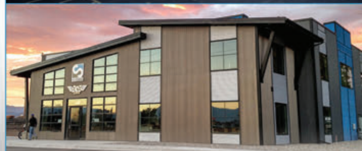
SCS Wraps - Bozeman
