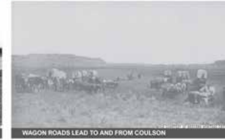
WAGON ROADS LEAD TO AND FROM COULSON
