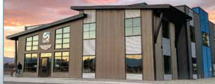
SCS Wraps - Bozeman
